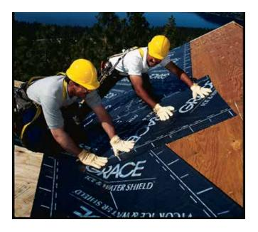
**Foldless release paper** – The foldless release paper provides multiple performance enhancements: fewer edge catches, 180° pull-back, ease of membrane cutting (single cuts) and membrane positioning, quicker "one-man installs" resulting in an easier, more productive release.
