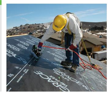
exposed for up to 6 months. It doesn't dry out or rot at high temperatures. It doesn't crack or become brittle at low temperatures.
